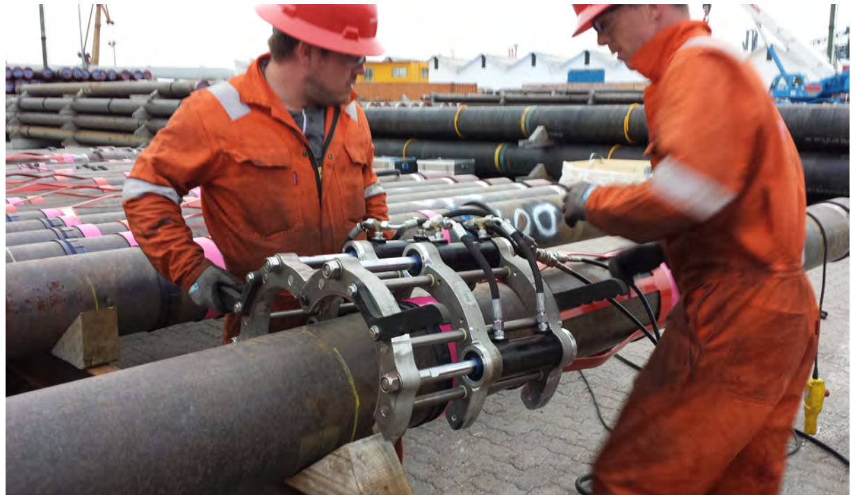
Installation of 13 5/8" UROS-CT and Ace Ratchet Collars (ARCS)
